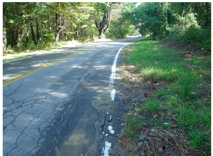
Sediment along a road side near a catch basin, indicated by a yellow arrow. Sediment is a carrier of both bacteria and nutrients.
