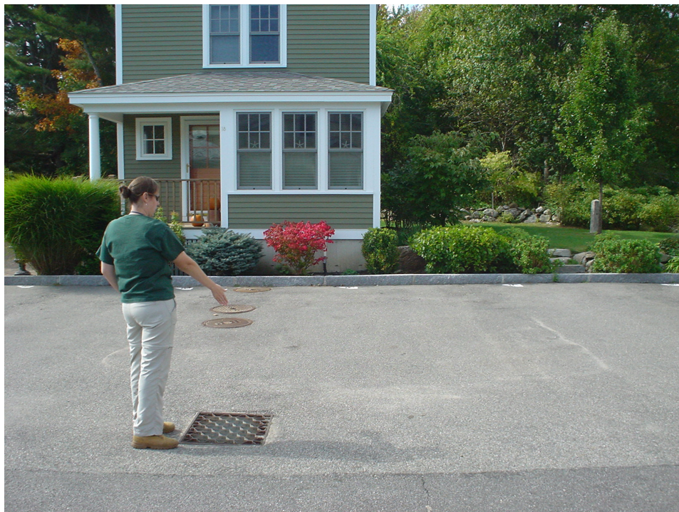
Storm drain in the parking area of a residential development that catches untreated area runoff.
