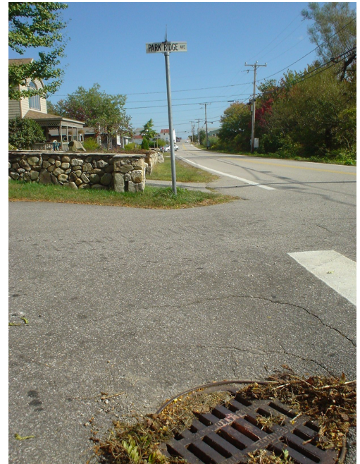
Catch basin with debris at the corner of Park Ridge Rd
