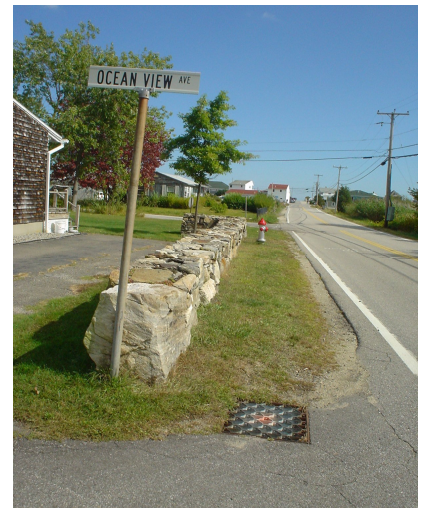
Catch basins collect stormwater that carries pollutants to Parsons Creek.
