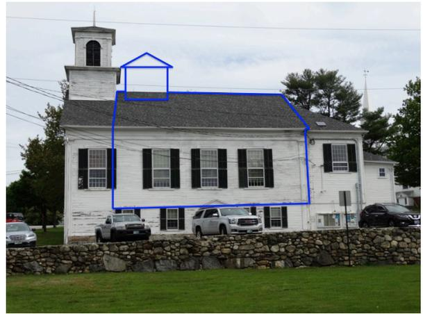
Figure 46: Annotated view of Rye Town Hall looking north, showing the proportions of the 1839 church within the current structure.
