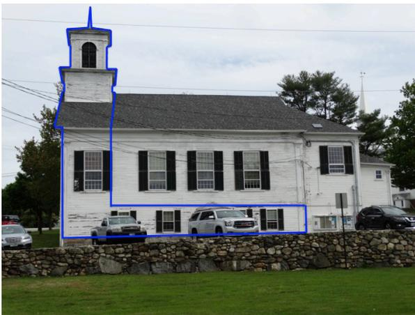
*Figure 52: Annotated image of the Rye Town Hall looking north, showing the lines of the ground-floor, front and tower additions made in 1873.*
